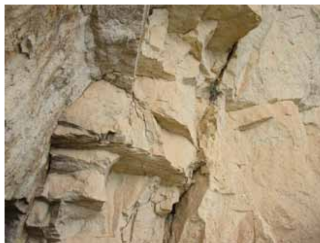
View of the base of the cliff. In this sector, angular blocks were detached with levers from the rock face by profiting from natural fissures.
