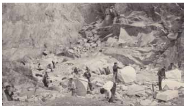
View of the fashioning conical oil rollers in the area of Gerena. The quarry is not identified. The quarry produced both conical oil rollers and rectangular blocks for construction (from Acuña Carabantes 2004).
