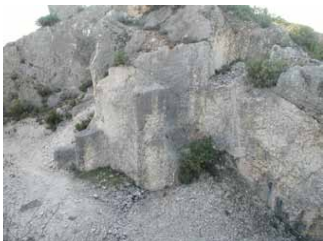
View of one of the working faces of the northern sector of the quarry where millstones were extracted on superimposed levels leaving diagonal pick marks.
