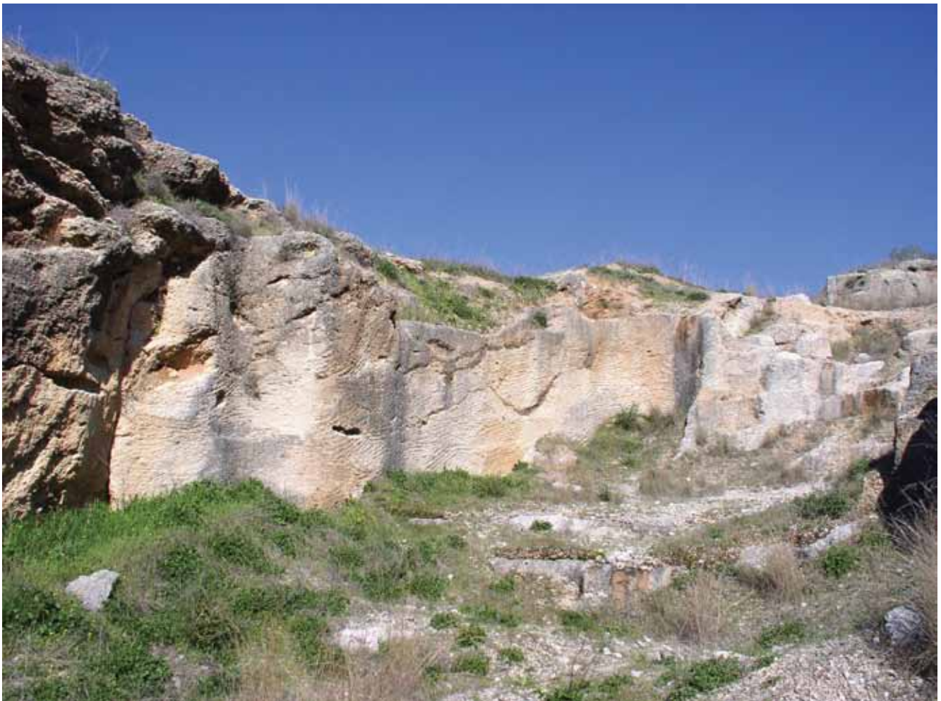
View of a quarry face in the north-western sector with high, tubular extraction hollows bearing multiple diagonal pick marks.
